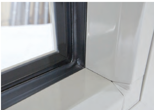
Down to the last detail: perfect design with glazing bead angles
